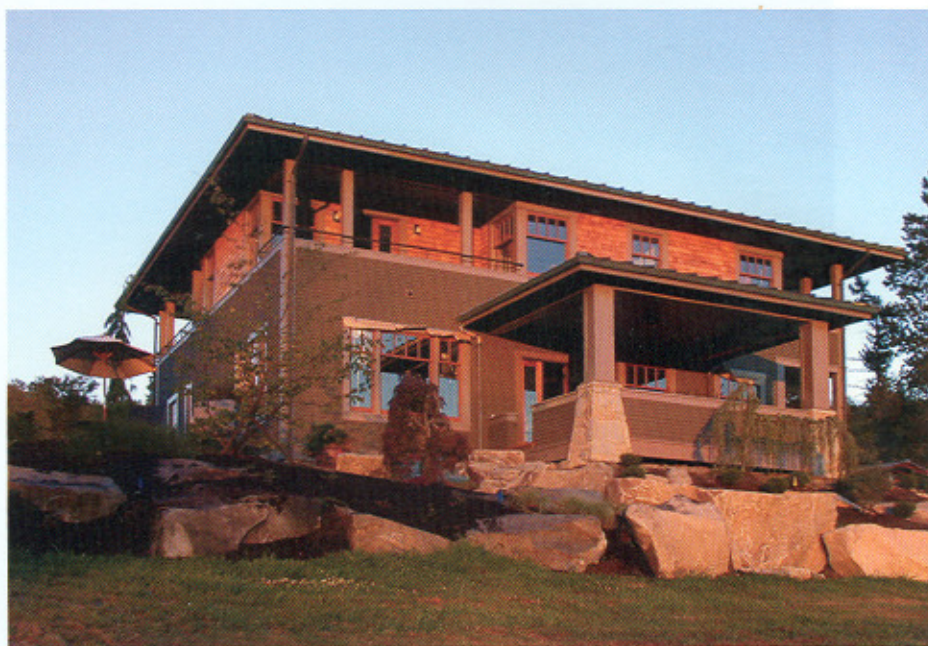
This house used stack framing which reduces the amount of wood used in framing by 25-30 percent while increasing insulation—all while lowering both material and labor costs. — Harrison Architects/ Anderson Builds; photo credit: Rob Harrison, AIA
