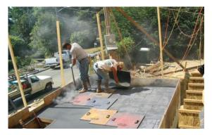
The Sensible House has a 7,000-gallon cistern that collects rainwater for landscape irrigation and toilet flushes. Its concrete lid — made with recycled fly ash — doubles as a patio.
