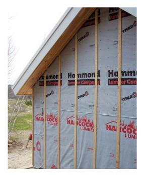
Taggart installs rain screens to keep water out of walls and prolong the life of trim, siding, and paint.
